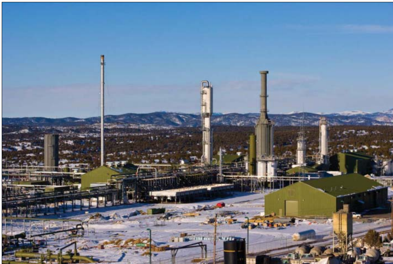
In March 2009, Enterprise Products Partners LP announced start-up of the expansion at its Meeker II gas processing plant in Colorado's Piceance basin. The expansion doubled capacity to 1.5 bcf/d with the capability to extract as much as 70,000 b/d of NGL. Enterprise expects gas volumes at the expanded plant to reach 1.1 bcf/d by yearend, when NGL production will reach 60,000 b/d. Photo from Enterprise.
